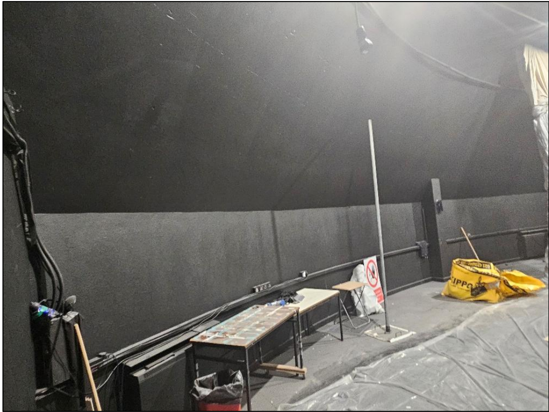
Plate 43 Walls and sloping roof require dry lining and insulation.
