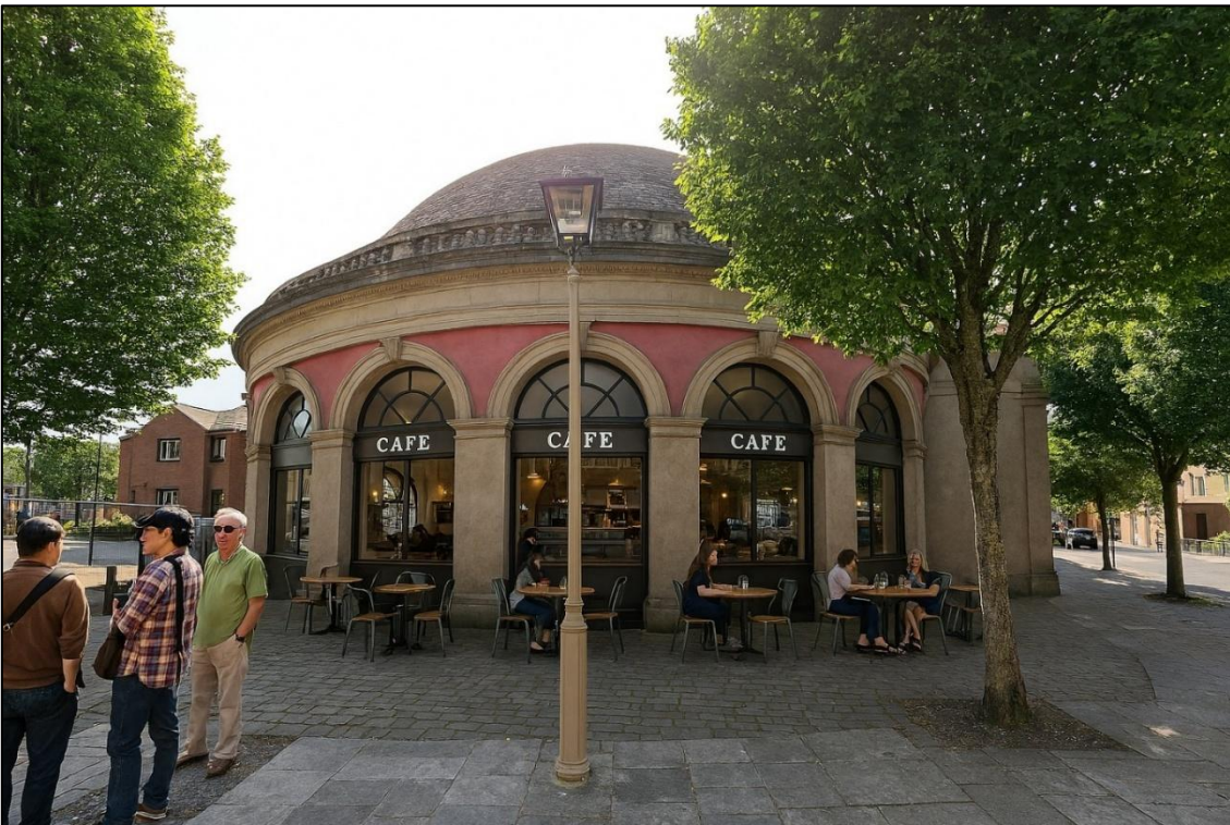
Plate 7 Opening up arches for cafe
