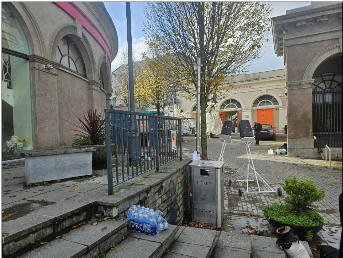
Plate 22 The entrance arrangement could be improved; it is unnecessarily complex with parked cars often obscuring the entrance and ramp beyond.
