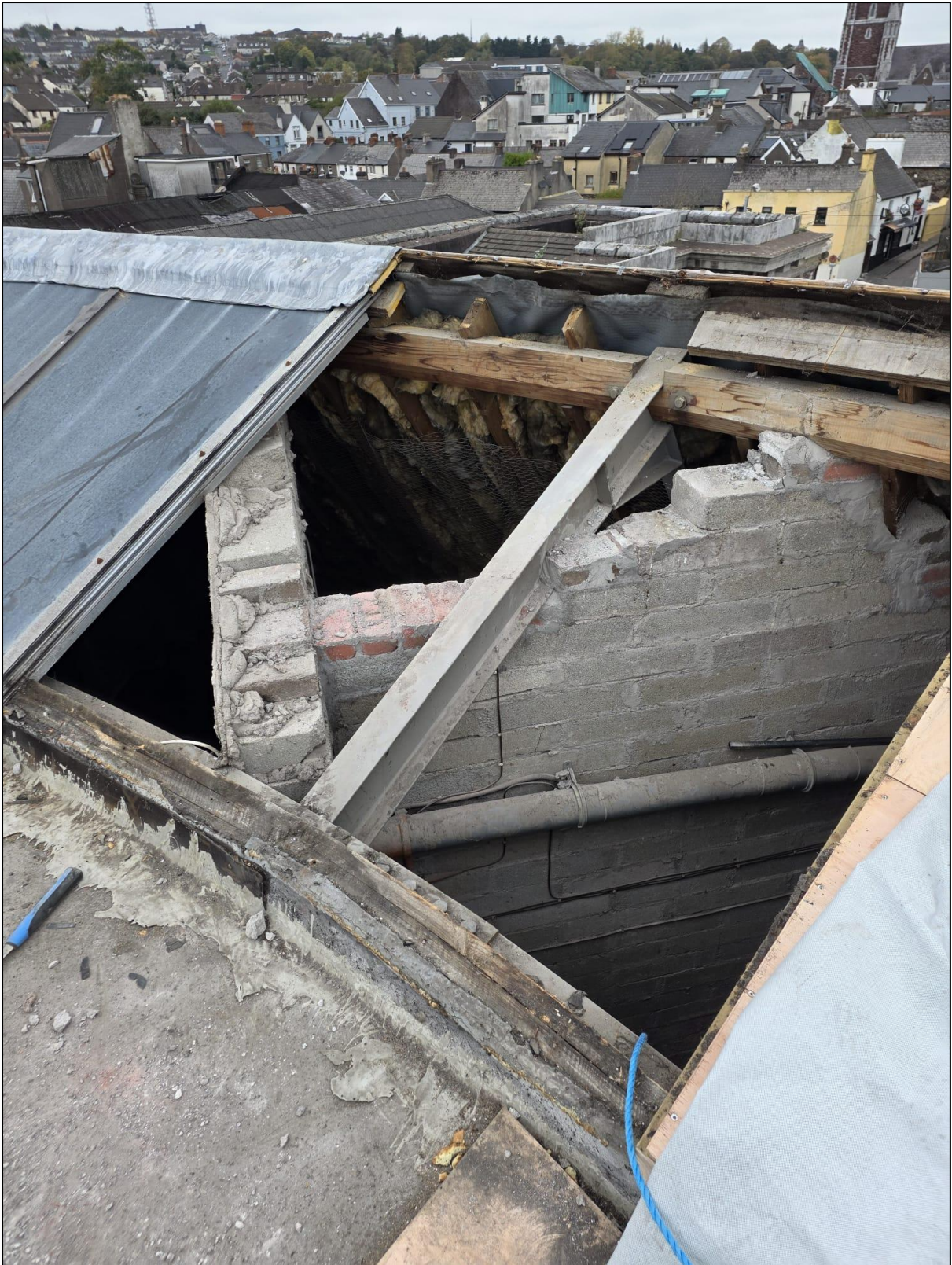
Plate 48 Walls are not sound proofed between rooms. Plate 49 Complex roof structure in good condition.
