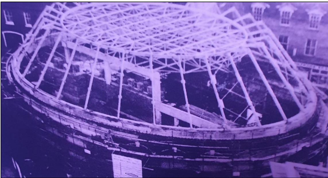
Plate 12 The spider like steel roof structure built during the 1980s during reconstruction after the fire. The central column is not used, a flat internal roof added and the roof pitch in increased.
