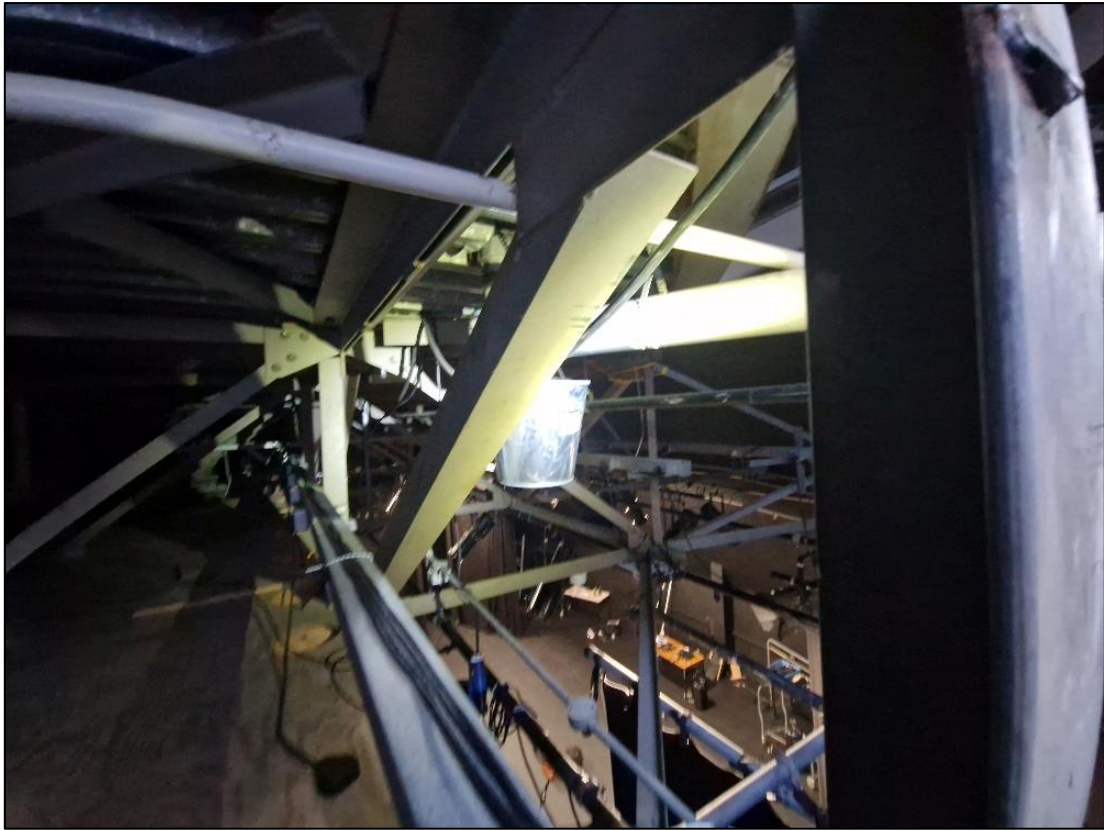
Plate 52 Complex roof structure in good condition.
