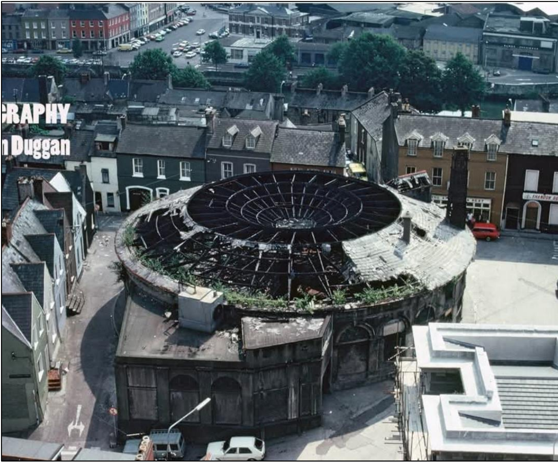
Plate 11 Photograph of Firkin Crane roof during the 1980s. Note the flat top course of the roof structure. Note also roof extension on the north elevation and the large chimney on the west, presumably a later addition. Bensons original radial roof structure of 32 radial trusses like a cartwheel is clearly visible where slates have been lost.
