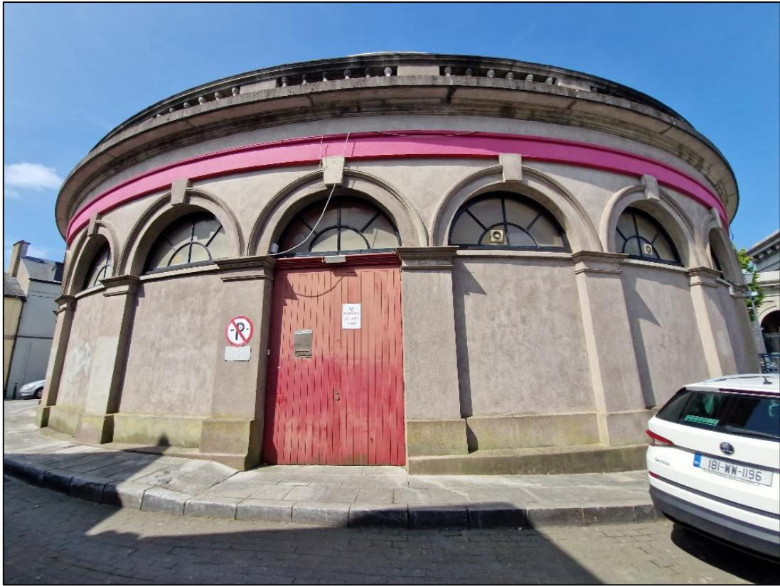
Plate 17 the original open arches of the Firkin Crane (Crane House) are now blocked up with non-structural masonry with a few door openings.
